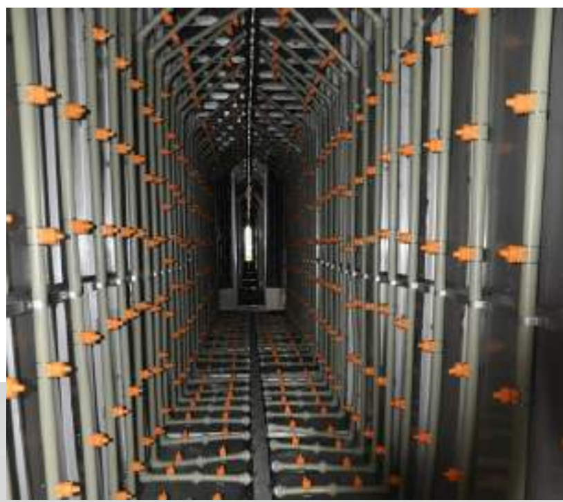
Surface Cleaning of The Metal Parts
